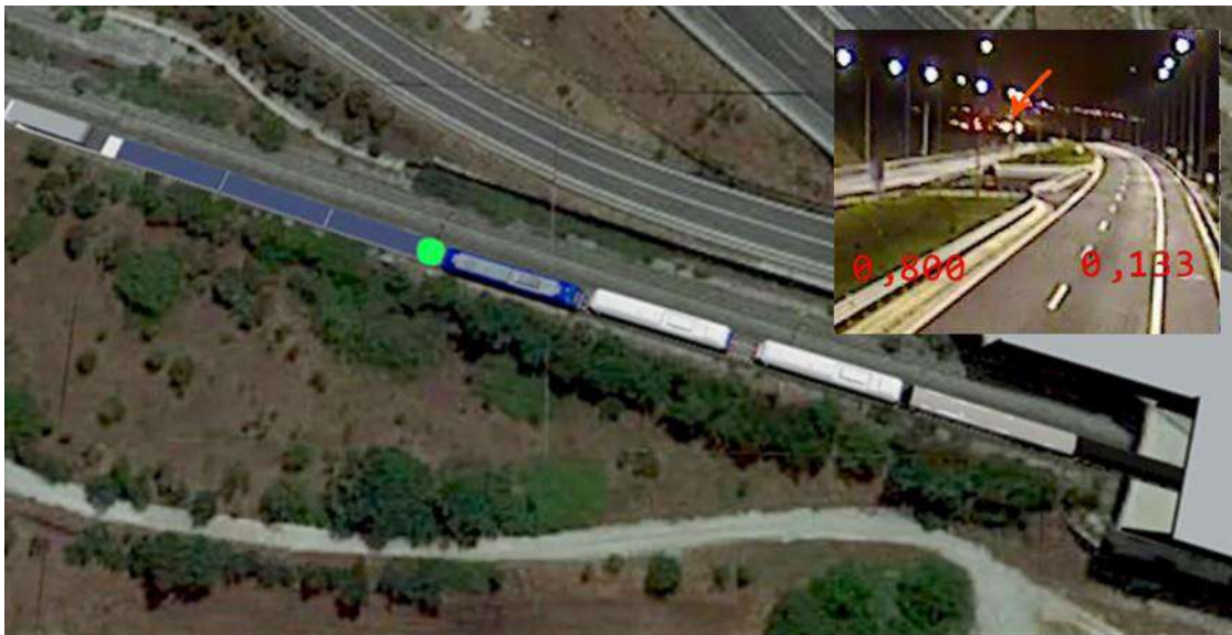
Figure 58. Estimated point of initial ignition.
