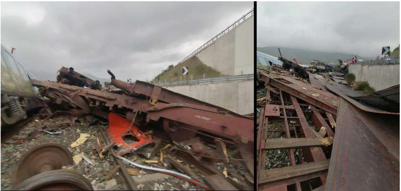
Figure 82. Platforms as found on the accident site.
